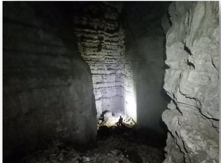
RAE 001 Sasule, clogged shaft
